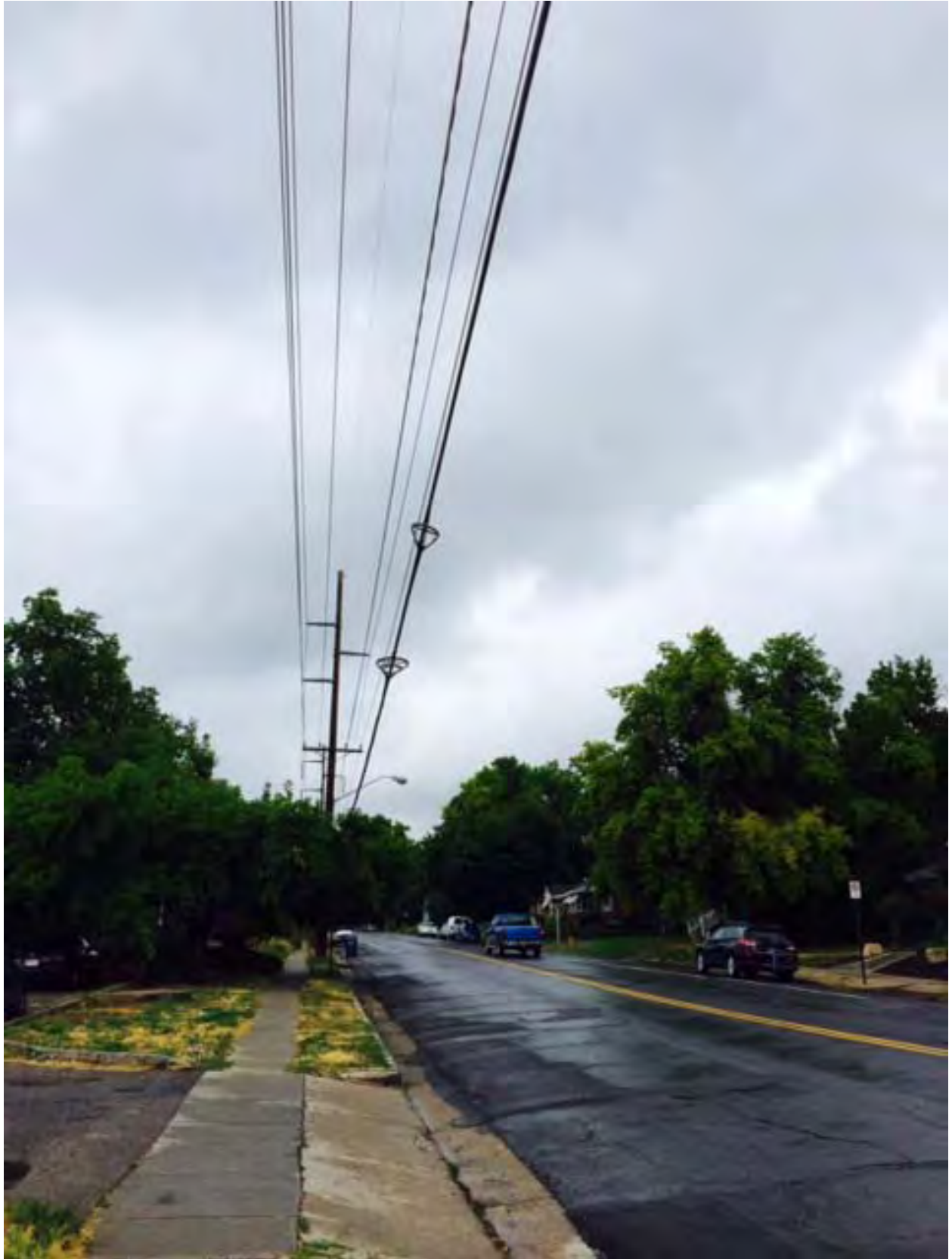
Photograph is looking towards the north along 1100 East. The utility pole that is proposed to gain additional wireless antennas is directly to the south of this location.
